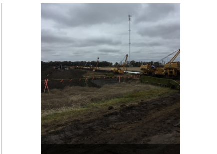
Description & Location: SSKP 907+833 Souris River HDD section Welders finishing up weld Side Booms holding pipe in place Facing northwest
