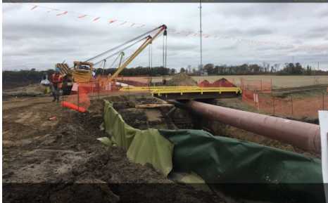
Description & Location: SSKP 907+833 Souris River HDD section Bridge complete pipe resting under bridge Very congested area stayed out of way Photo facing northwest
