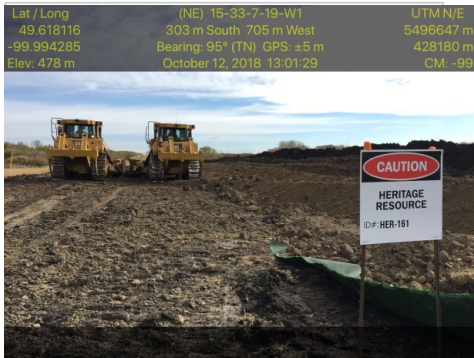
Description & Location: SSKP 885+020 Heritage Resource area HER-161 Dozers working together stripping Cultural monitors assessing area Facing east
