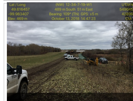
Description & Location: SSKP 886+260
