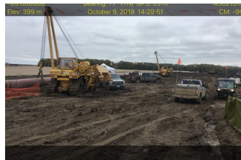
Description & Location: SSKP 907+833 Souris River HDD section Welders finishing last weld for section Side Booms holding pipe Photo facing northeast
