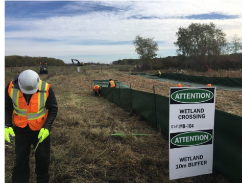
Description & Location: SSKP 885+250 Seasonal Marsh Class 3 MB-104 Installing wetland ramps Cultural monitor to the left Facing east
