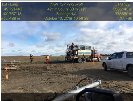
Description & Location: SSKP 827+700
