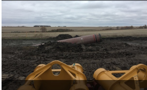
Description & Location: SSKP 899+860 Black Creek HDD section Pipe from bore sticking out of ground East of Black Creek Photo facing north
